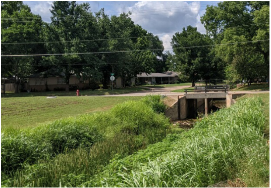
CREEK WITH STEEP EMBANKMENT
