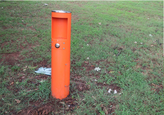
WATER BOTTLE FILLING STATION
