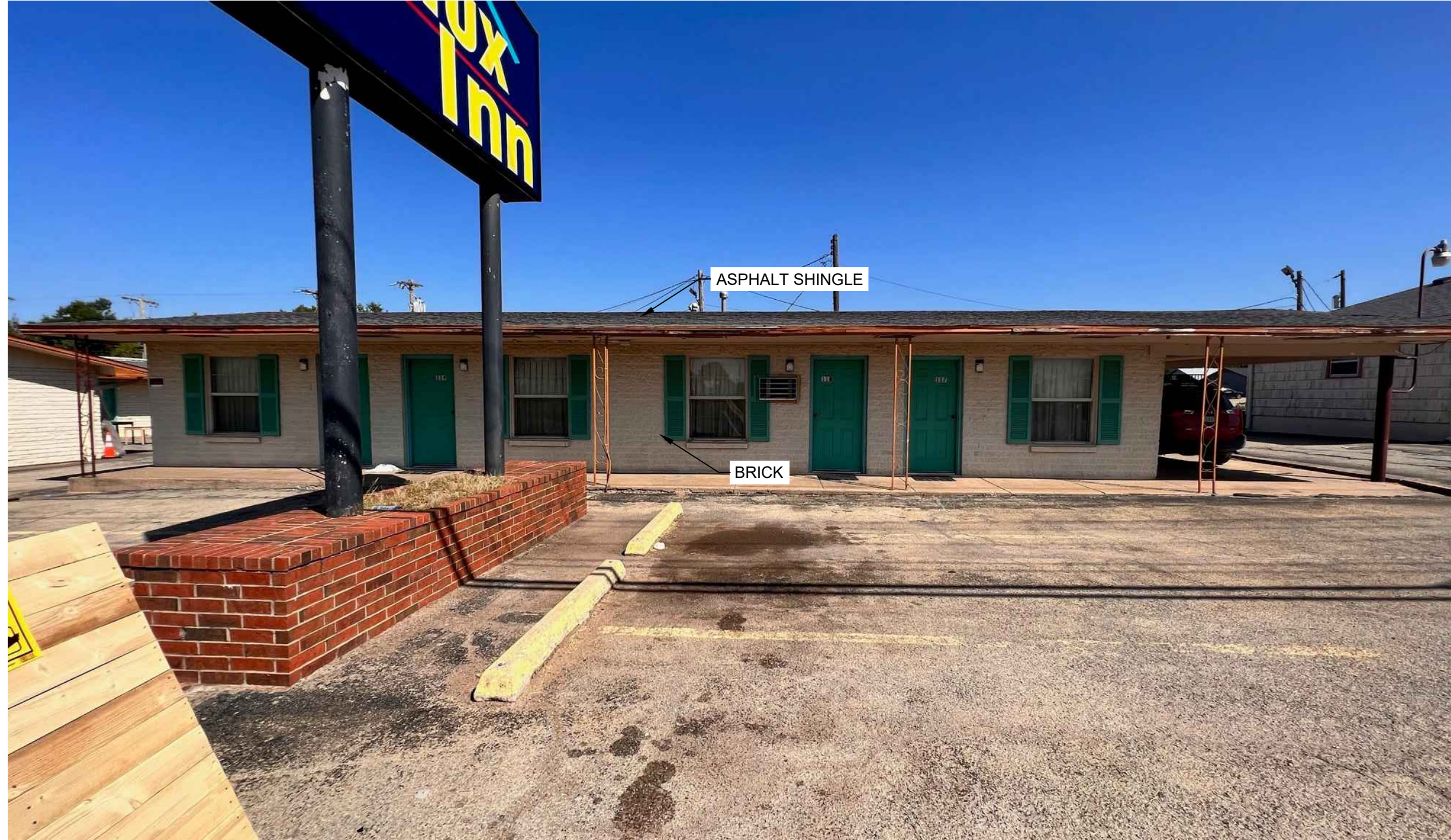
BUILDING 3 SOUTH FACADE
