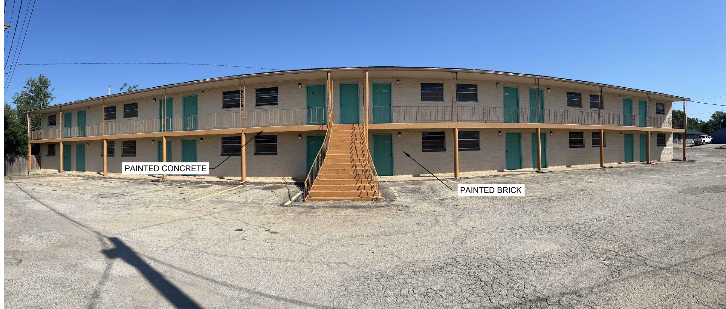
BUILDING 1 TWO STORY SOUTH FACADE
