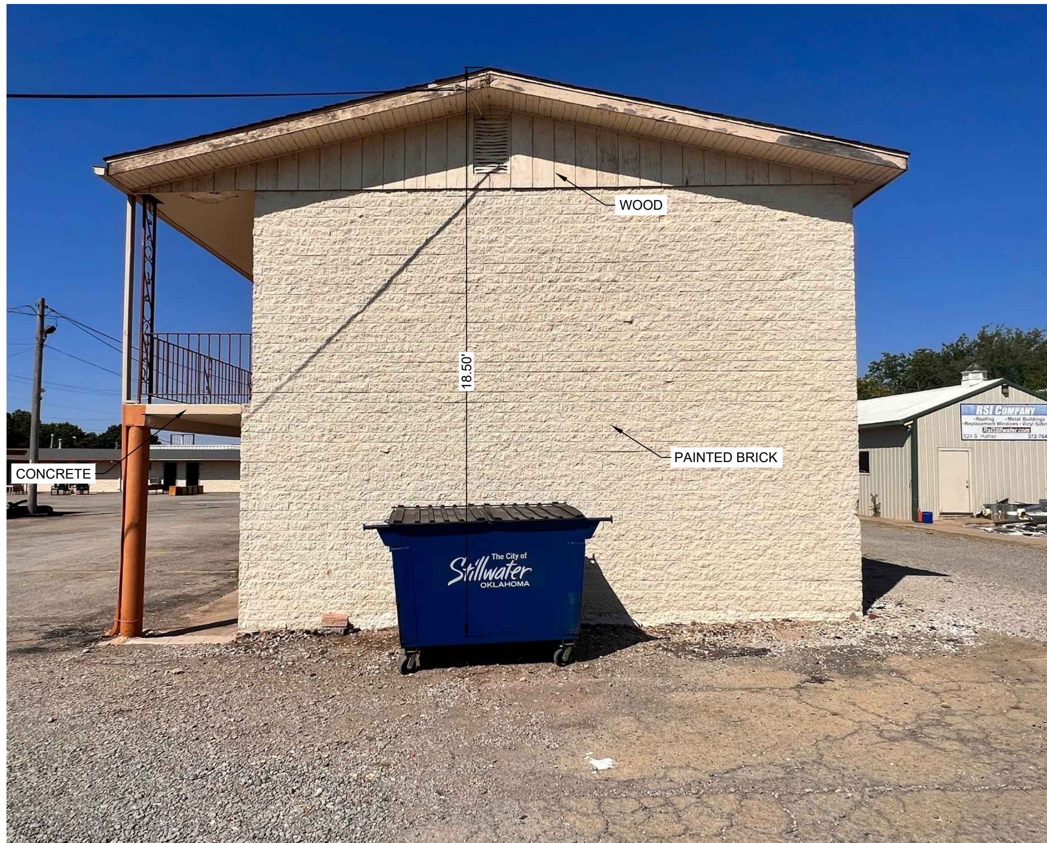
BUILDING 1 TWO STORY EAST FACADE
