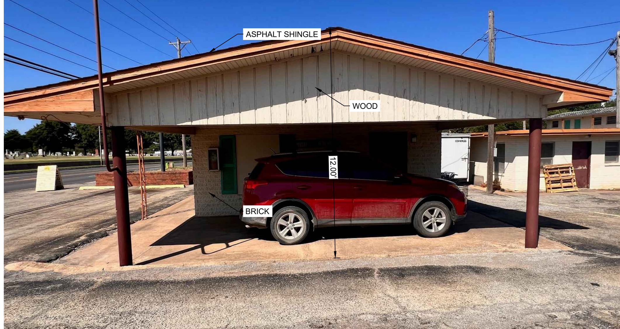
BUILDING 3 EAST FACADE
