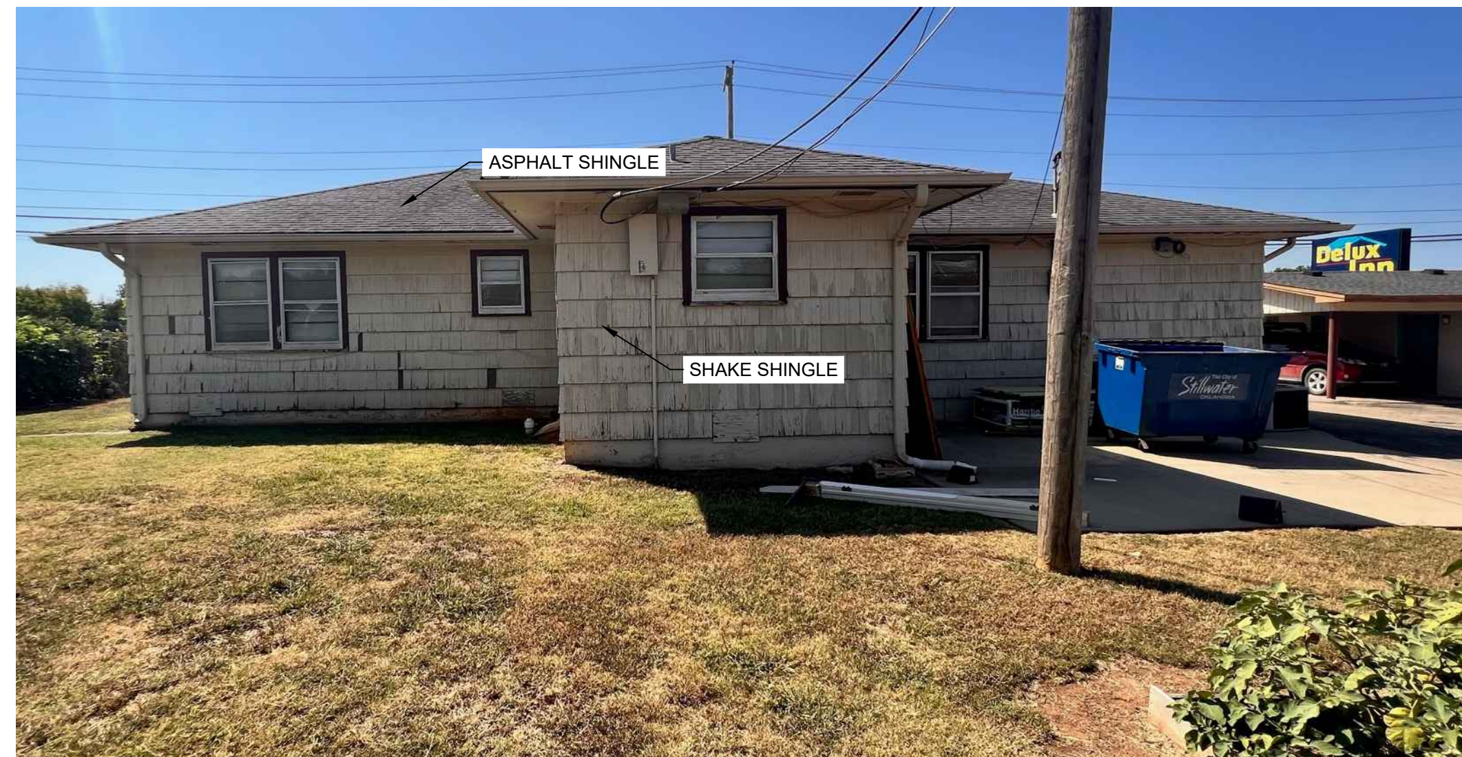
BUILDING 5 NORTH FACADE
