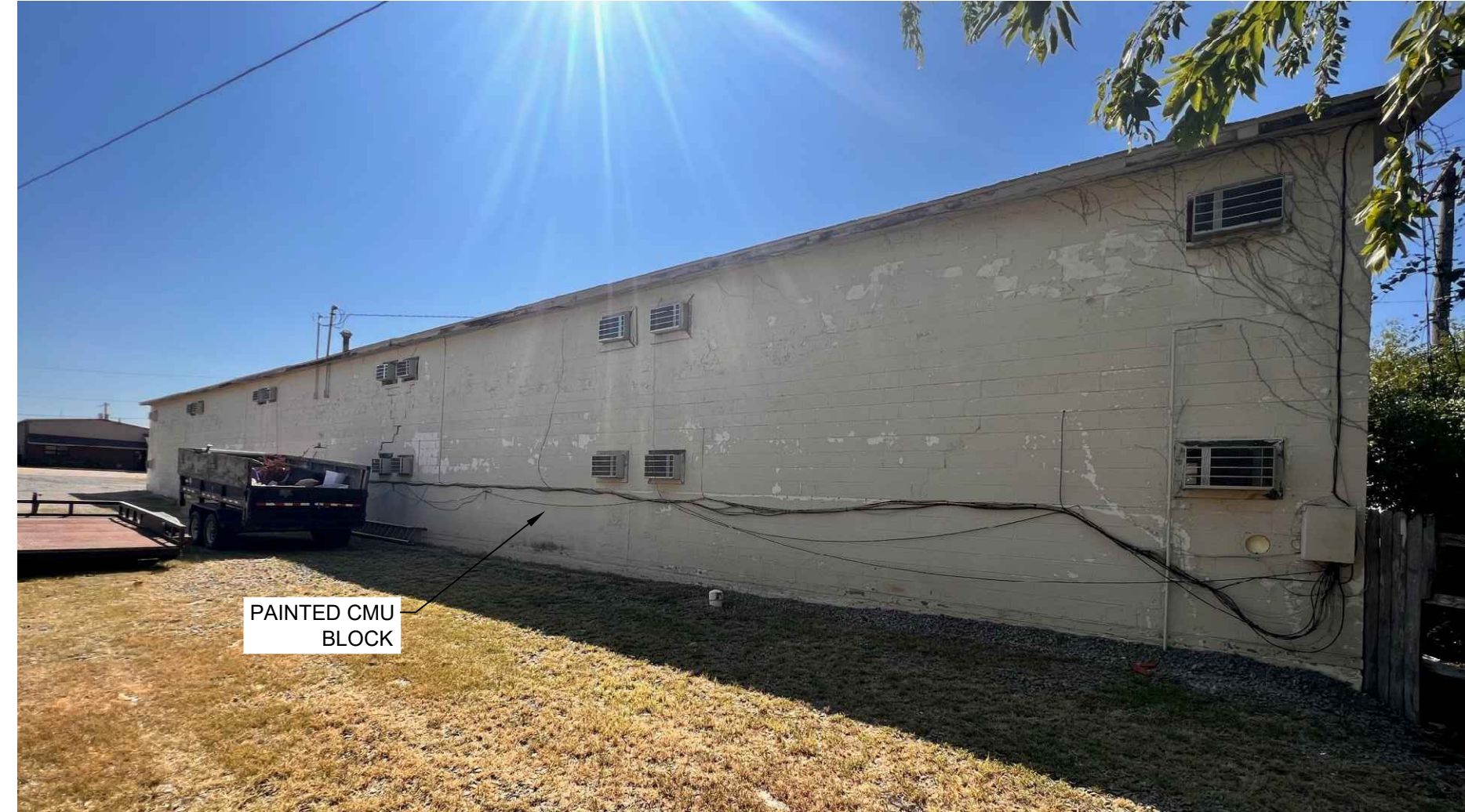
BUILDING 1 TWO STORY NORTH FACADE
