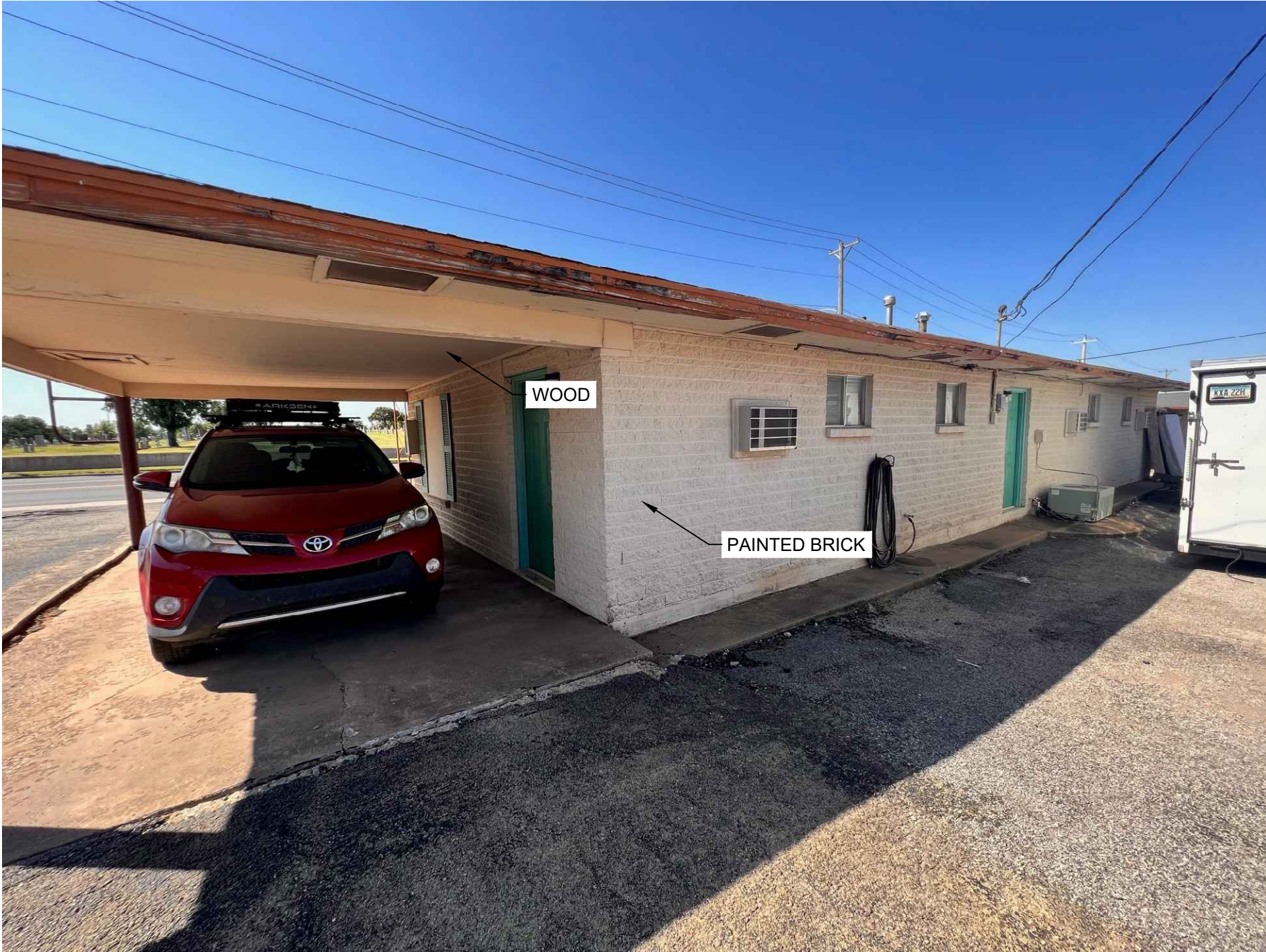
BUILDING 3 NORTH FACADE
