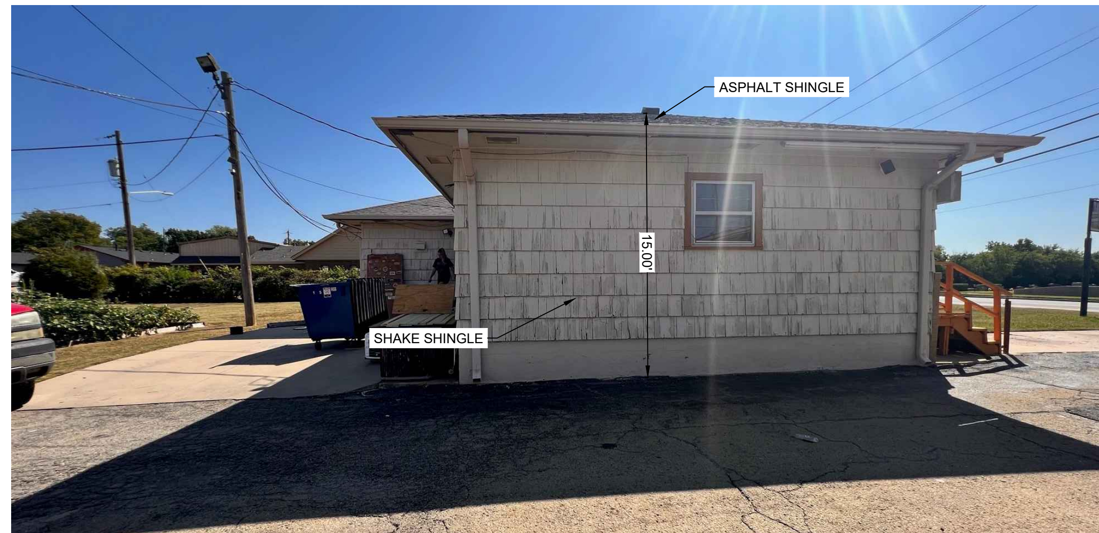
BUILDING 5 WEST FACADE
