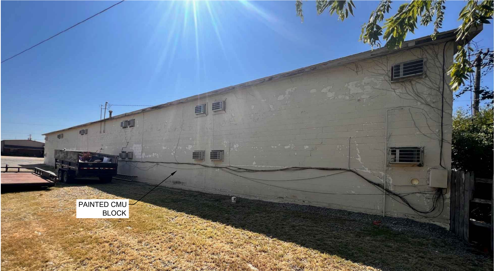
BUILDING 1 TWO STORY NORTH FACADE
