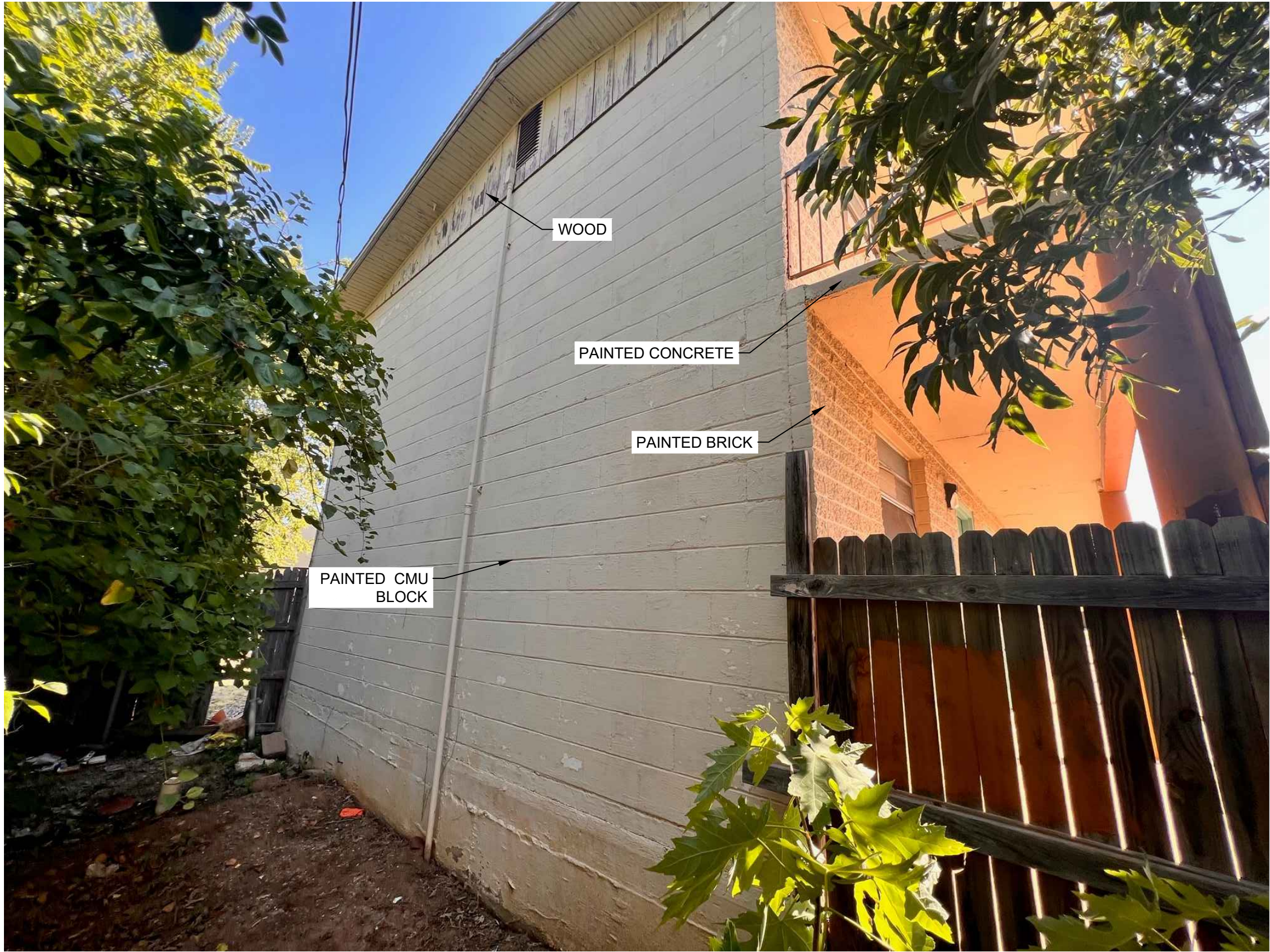
BUILDING 1 TWO STORY WEST FACADE
