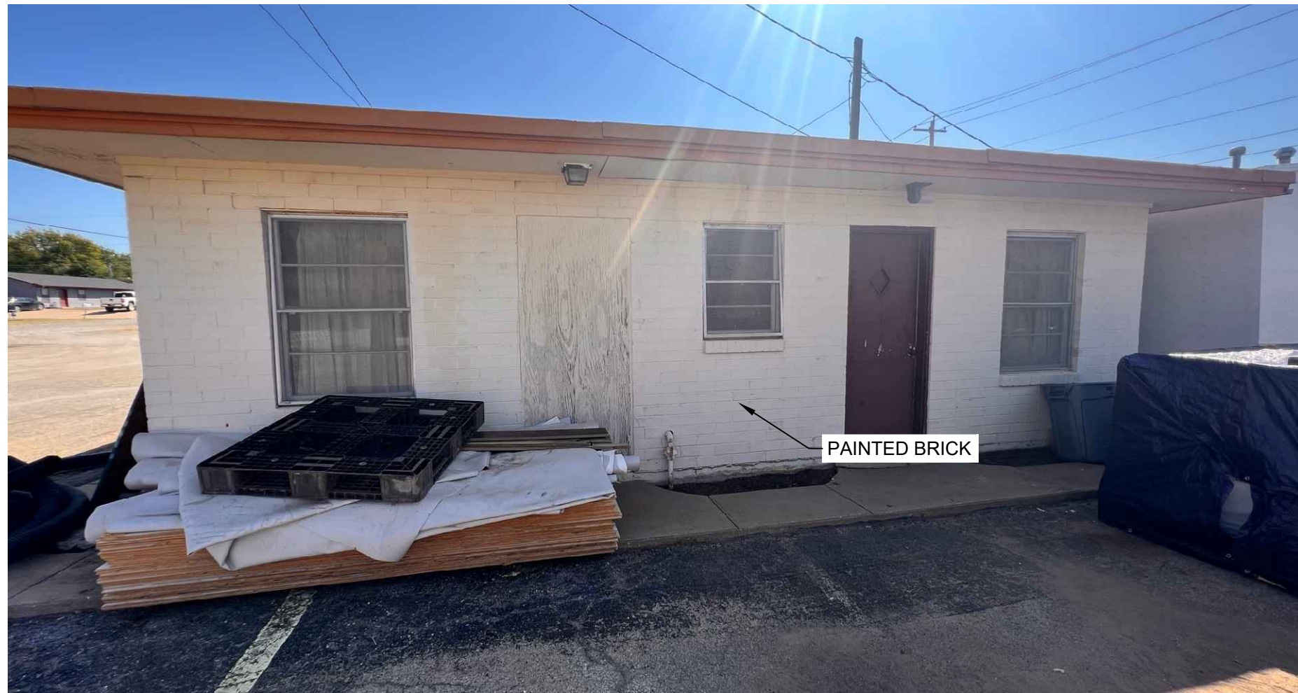
BUILDING 4 WEST FACADE
