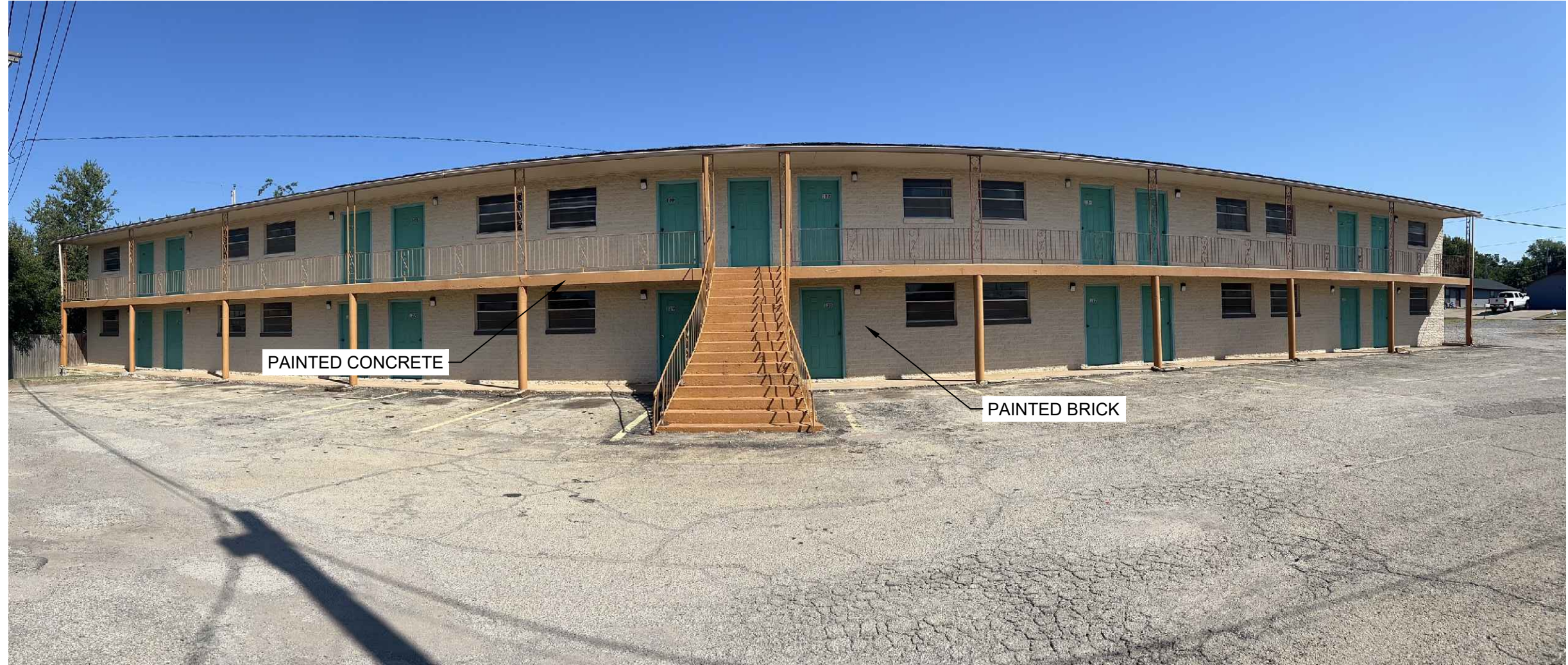
BUILDING 1 TWO STORY SOUTH FACADE
