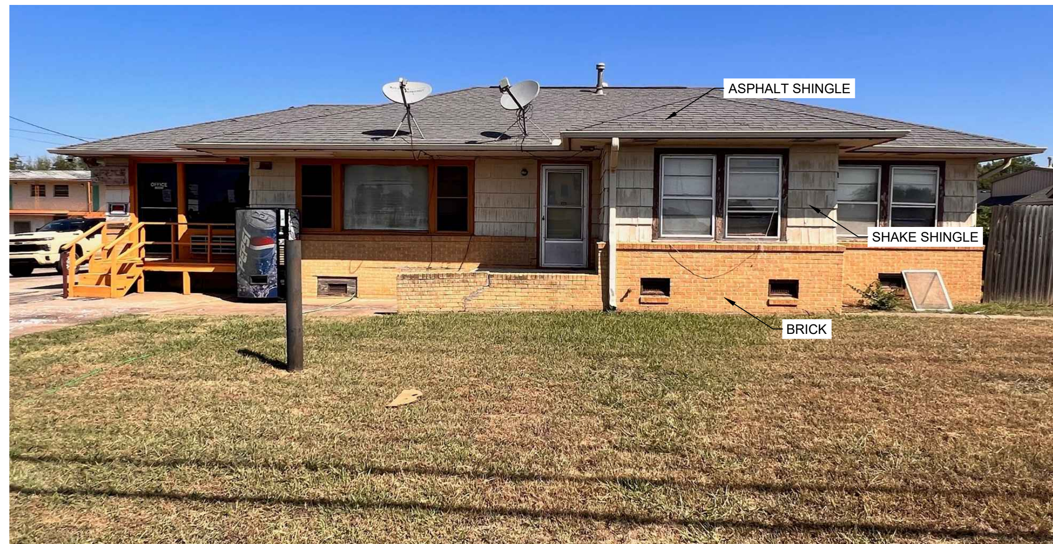
BUILDING 5 SOUTH FACADE
