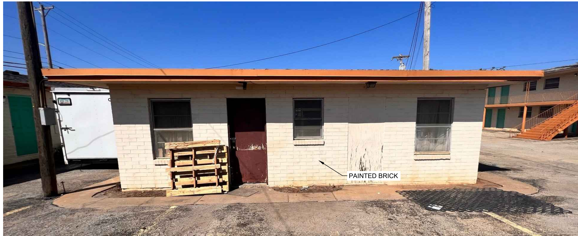
BUILDING 4 EAST FACADE
