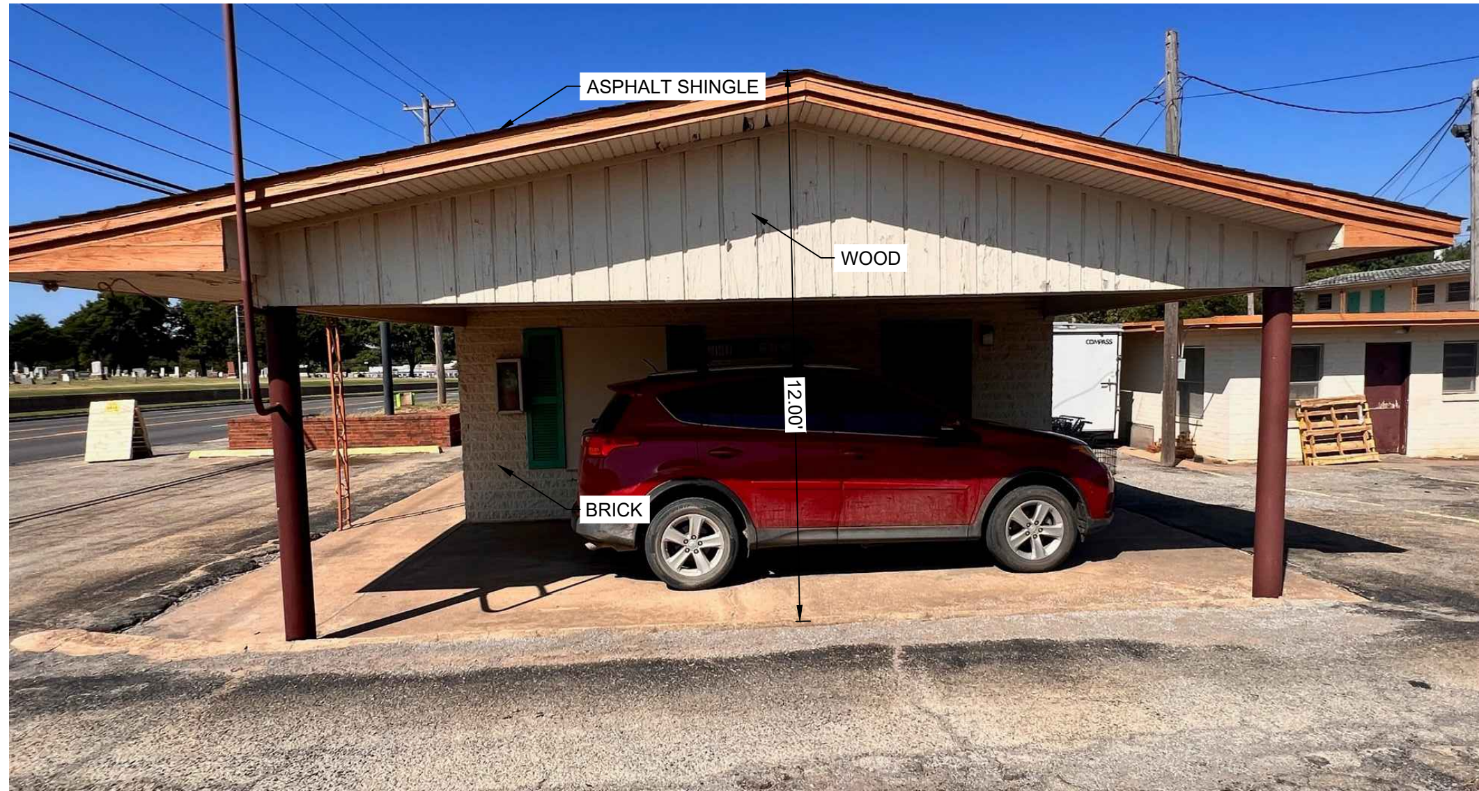
BUILDING 3 EAST FACADE
