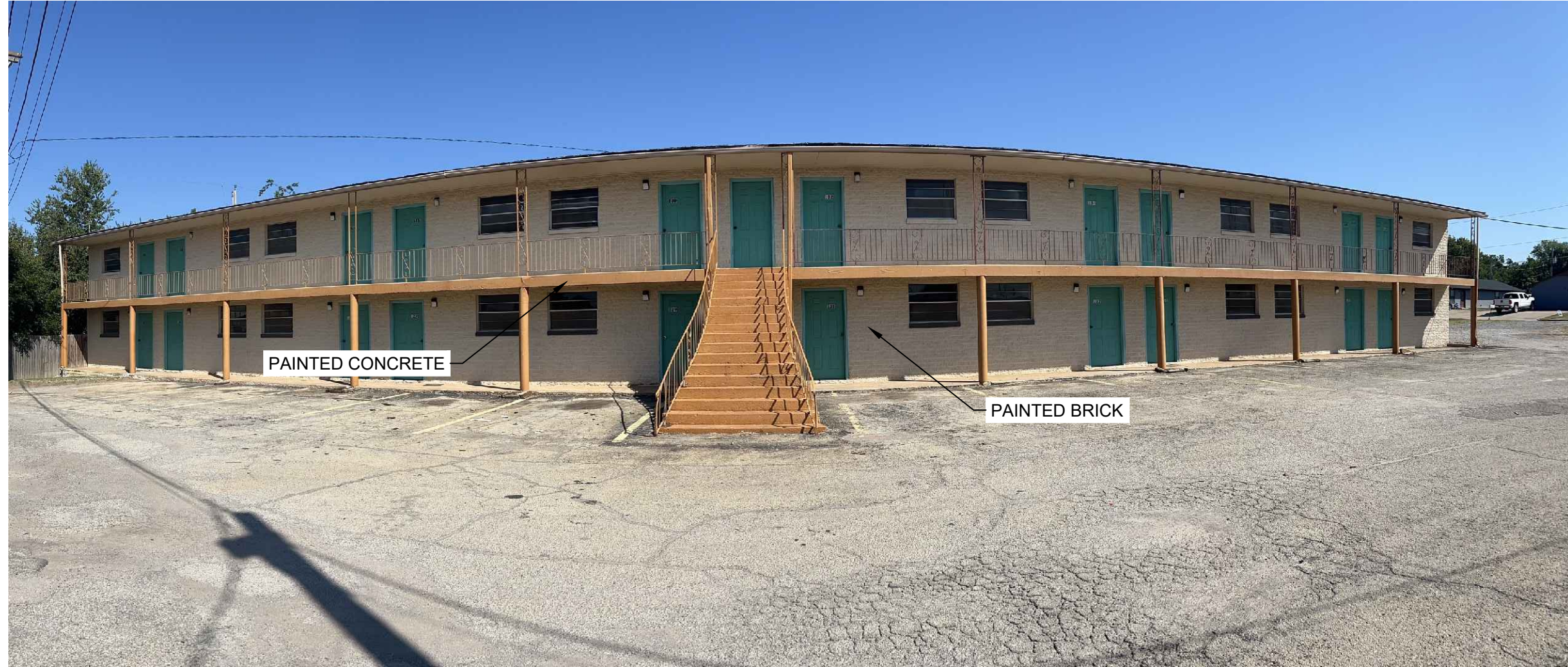
BUILDING 1 TWO STORY SOUTH FACADE
