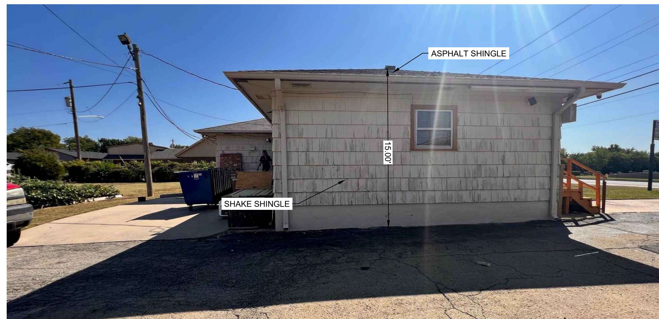
BUILDING 5 WEST FACADE
