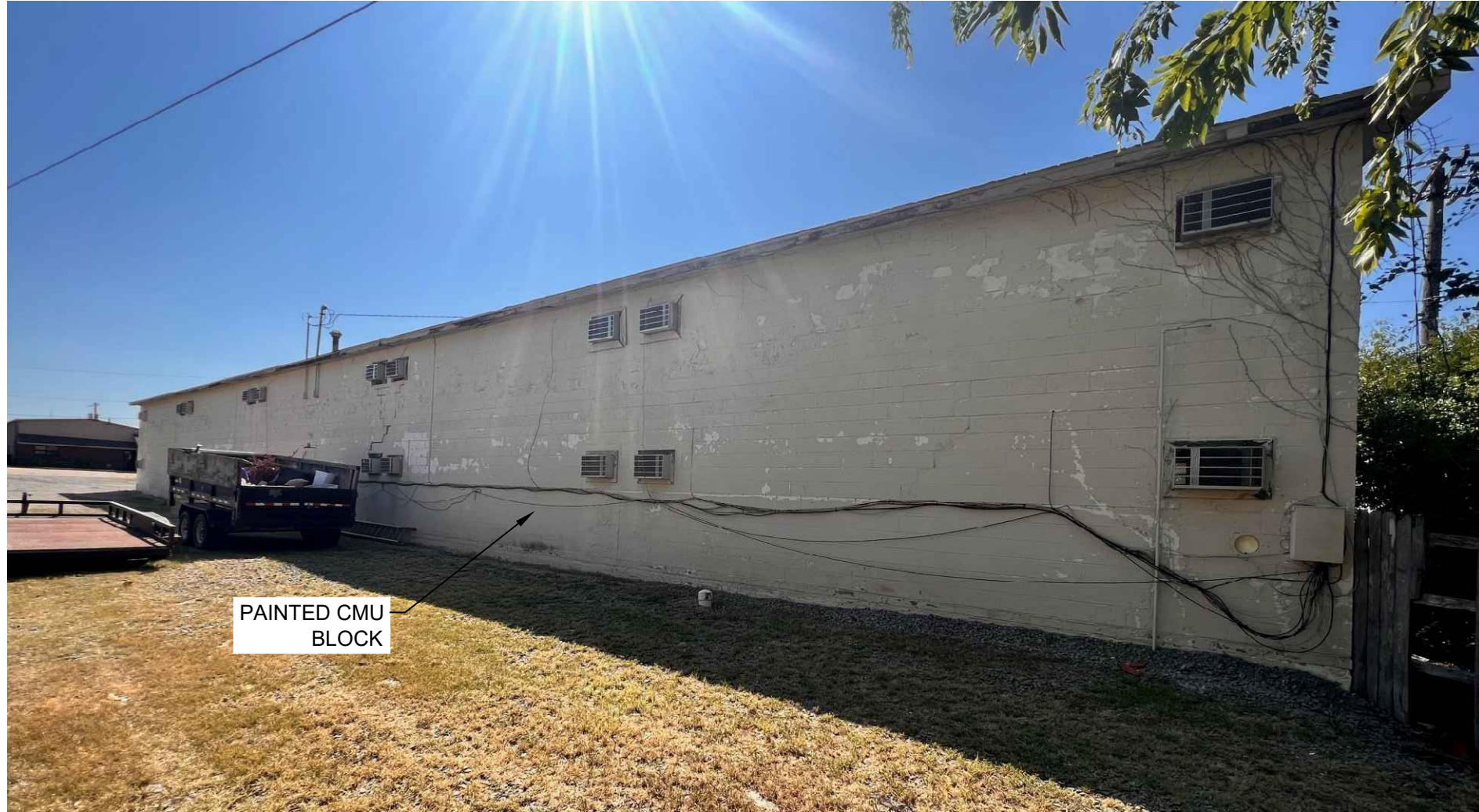
BUILDING 1 TWO STORY NORTH FACADE
