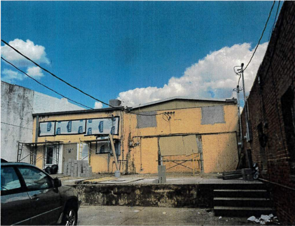
918-920 ALLEY VIEW AS REMODEL STARTS
