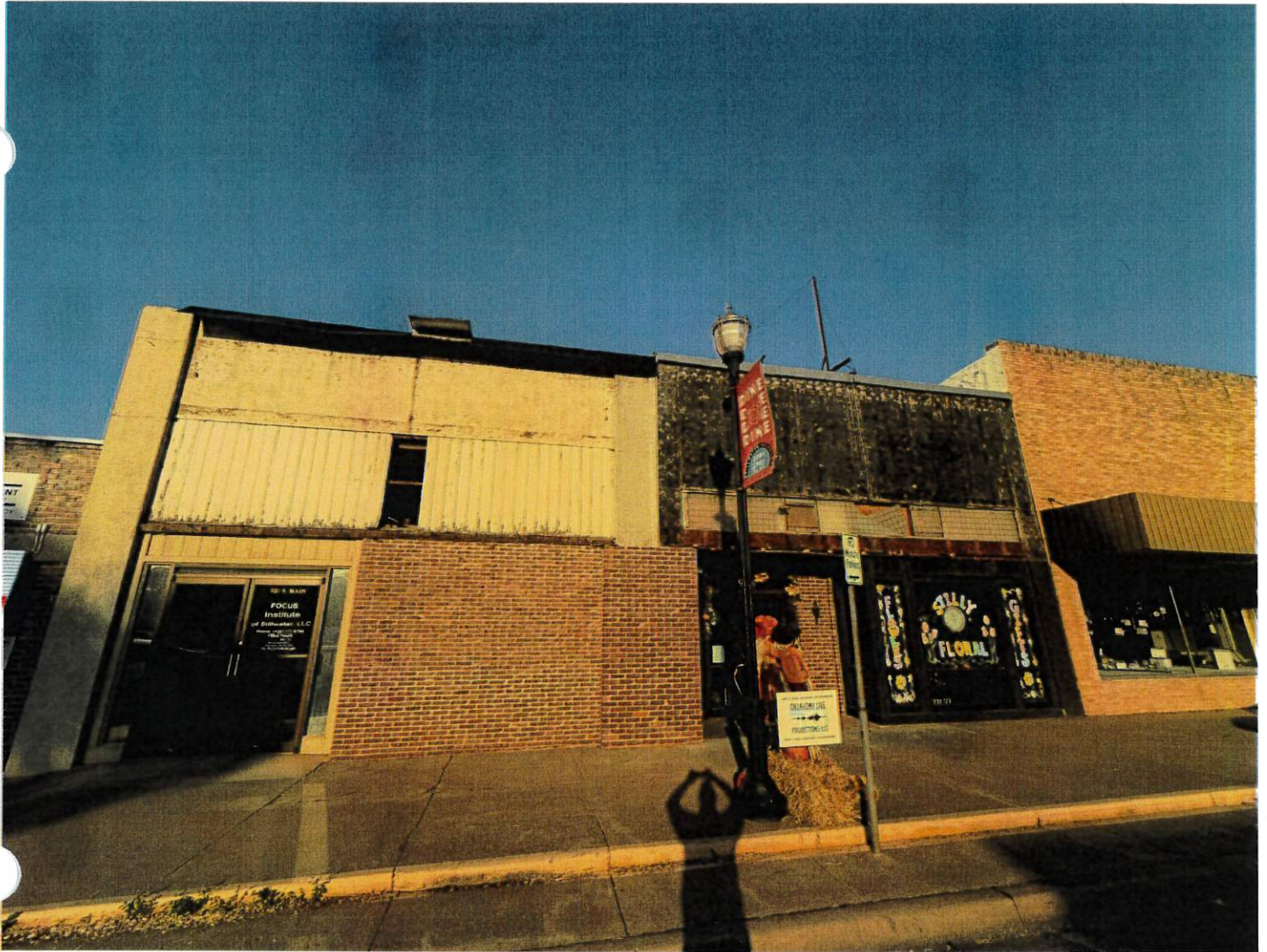
918 AND 920 AFTER THE REMOVAL OF THE MANSARD CANOPY
