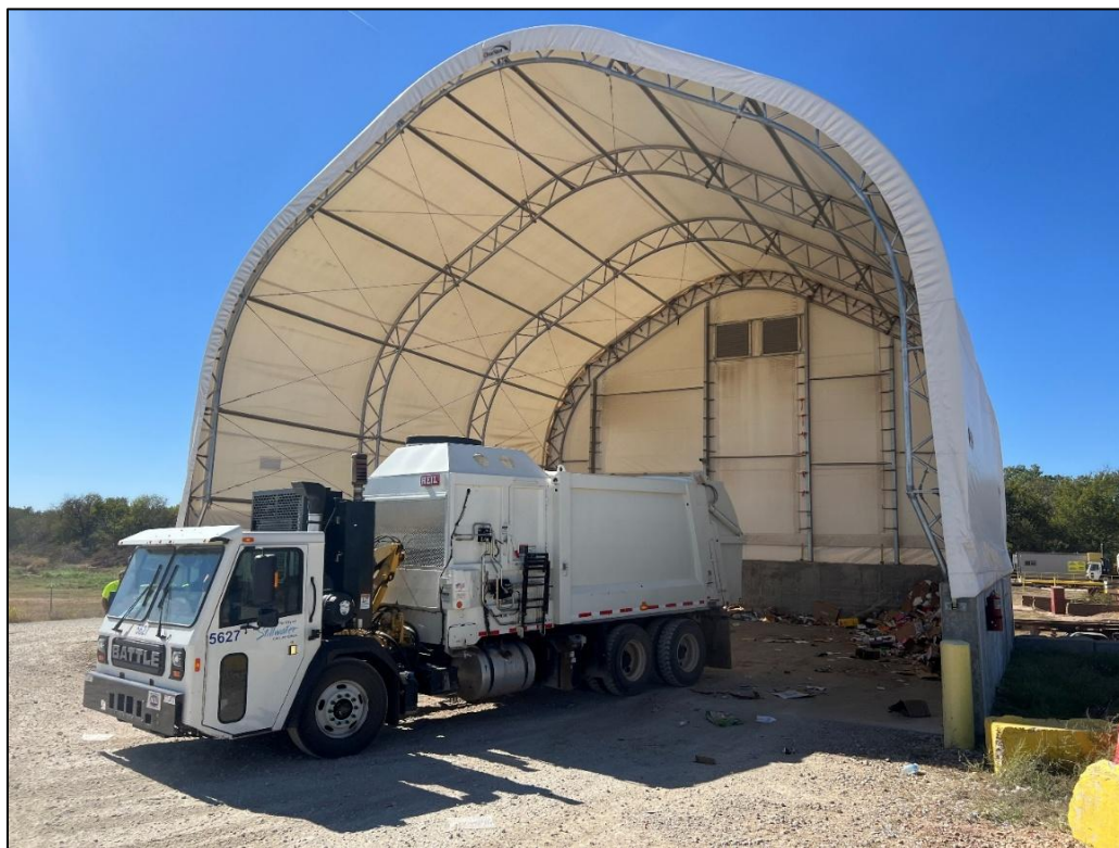
Figure 3-3 Republic's Recycling Staging Facility
