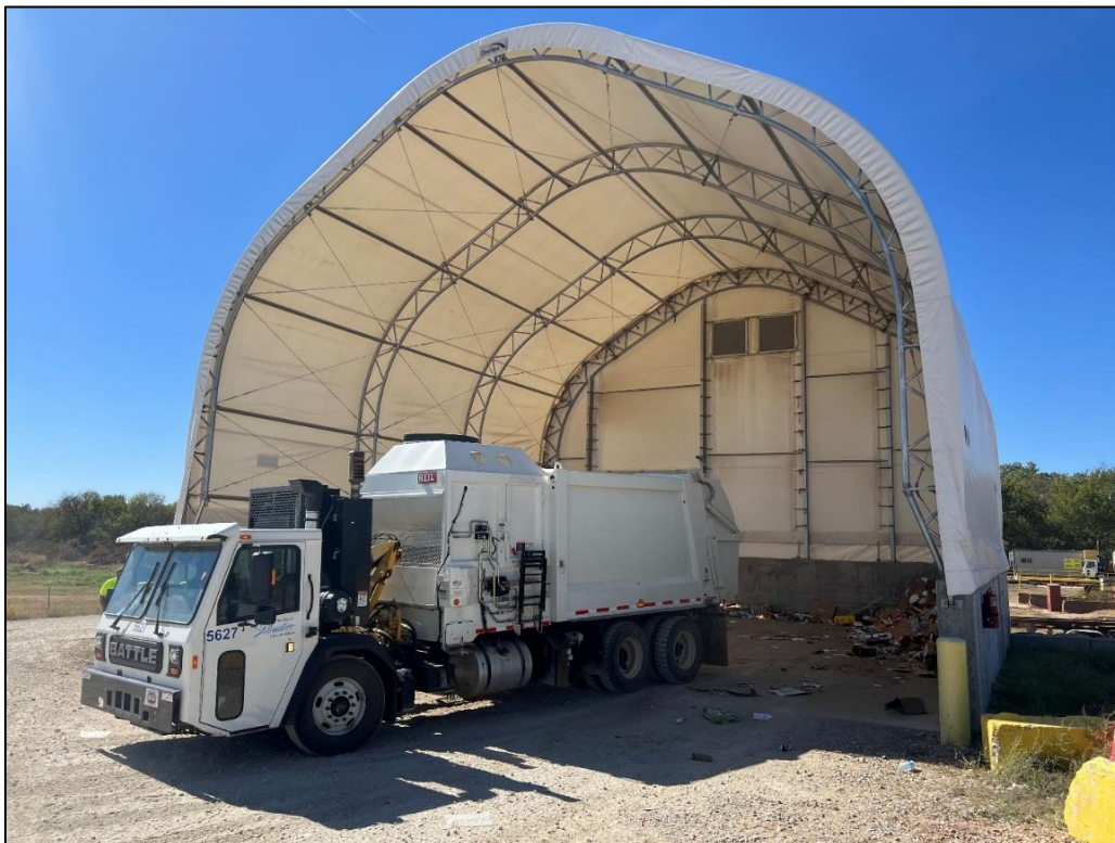
Figure 3-3 Republic's Recycling Staging Facility
