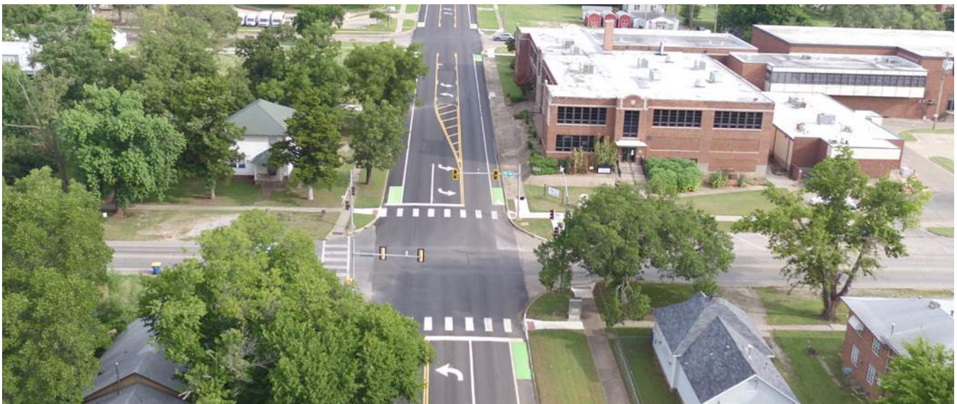
A multimodal intersection making use of left-turn lanes at W 9th Avenue and S Duck Street
