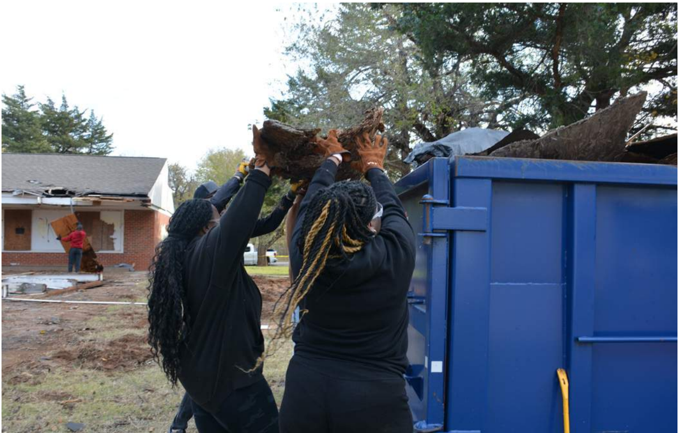
Washington school renovation, community volunteers.
