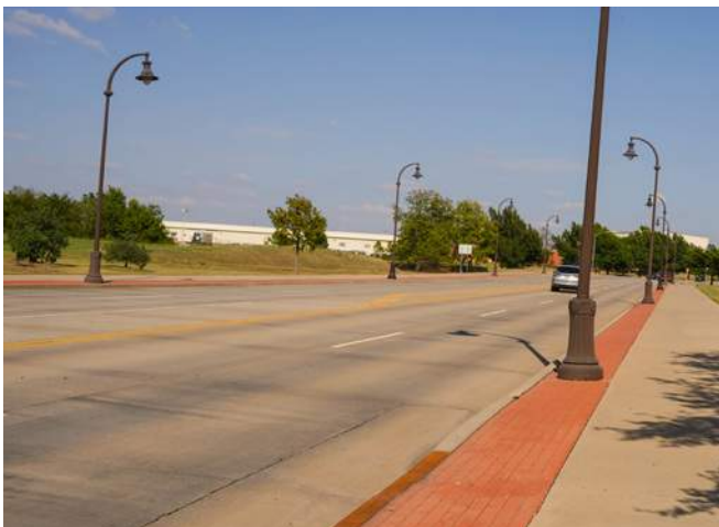
A major arterial class road in Stillwater.
