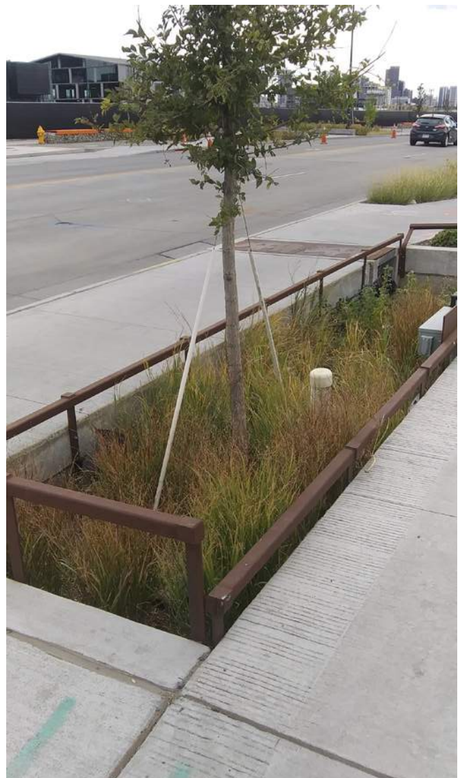
Innovative stormwater management, such as this bioswale, both contributes to the streetscape and can improve community resilience during storms and flooding events
